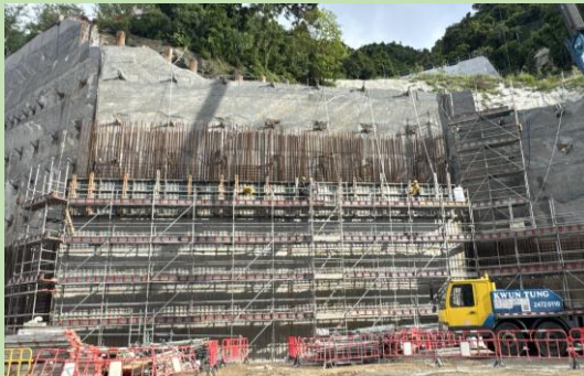
擋土牆混凝土結構工程 Concreting Works for Retaining Wall
